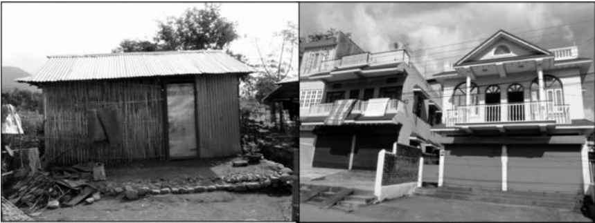
Fig. 4. Left: House for Family of Three along the Seuti Khola River; Right: Characteristic House of Retired British Army Recruits. Photos: Sudmeier-Rieux (2009).
